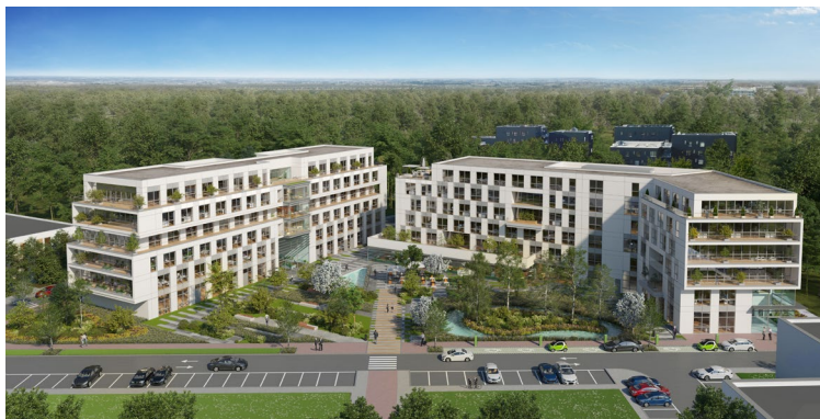
Eiffel Orsay Campus - 1 st phase of 13,500 m 2
